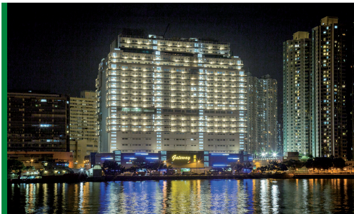
Gateway ts operates round the clock to cope with the international and other operation needs of its tenants. In the picture: The iconic outlook of Gateway ts at nights.
