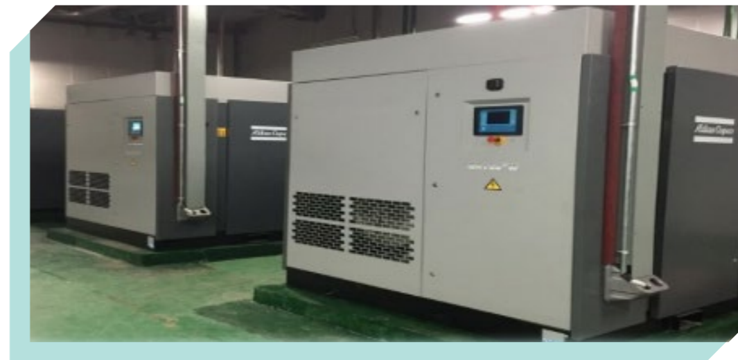
High-efficient air compressors at TCL Liquid Crystal Industrial Park
