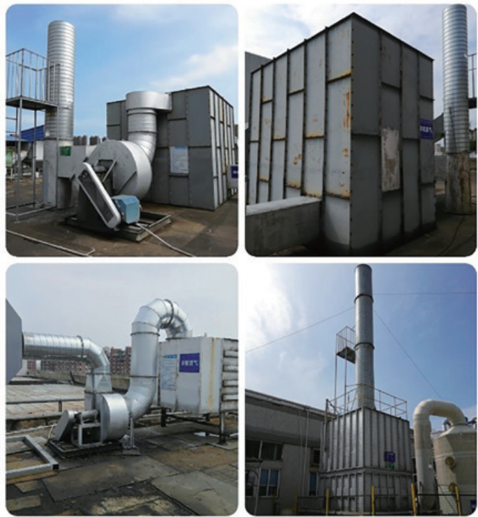
Activated carbon absorption devices at each discharge outlet within production plants 廠房內各廢氣排放口的活性炭吸附裝置
