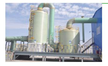
In order to control the phenylacetic acid generated from fermentation factories and the peculiar odor released from phenylacetic acid recycling process, the Inner Mongolia Company adopts the "cooling + alkali spraying + carbon fiber absorbing" and other treatment processes to effectively prevent peculiar odor from dissipation.
