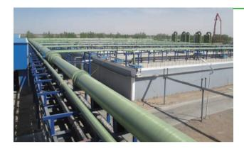
For the exhaust gas with peculiar smell generated in sewage treatment process, the factories adopt sealed collection measure on the odor source. The collected exhaust gas is deodorized through the process of "multi-level alkali spraying + ozonation" to reduce the impact on the surrounding environment.
