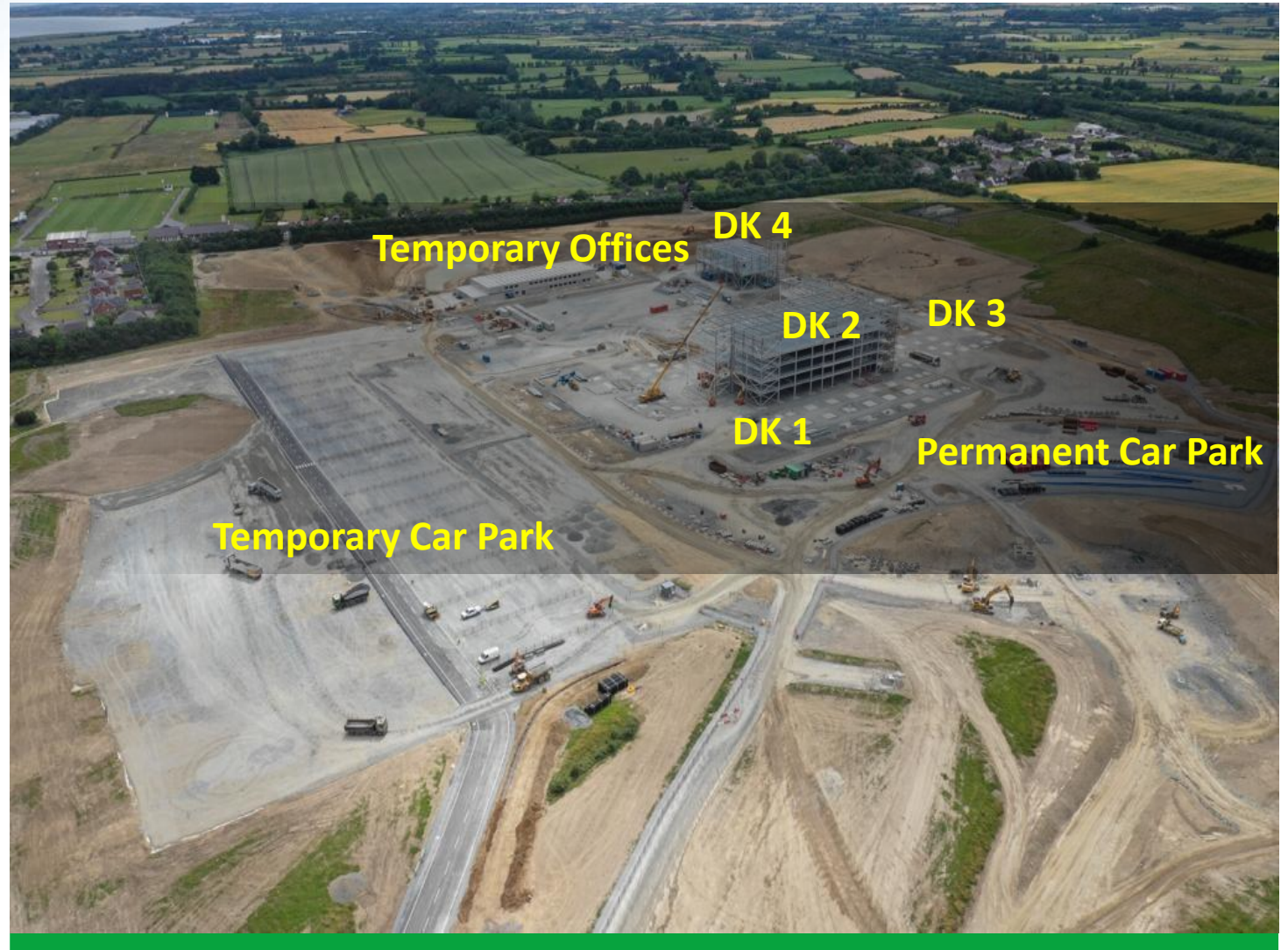
July Site Progress Photo
