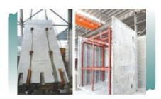
Precast elements construction system is widely adopted in our construction sites. As they are prefabricated in mass volume off-site, the volume of in-site concrete could be substantially reduced, which means the associated pollution generated in the course of concreting can be either reduced or saved. In one of our active construction sites, over 6,500 trees have already been saved through prefabrication adoption.
