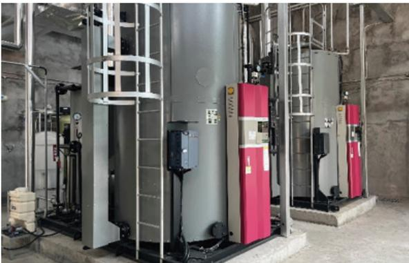
Low-NO<sub>x</sub> combustion boilers
